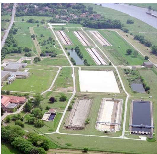
Figure 1. Aerial photograph of Hosterwitz water works for Dresden, Germany (©DREWAG NETZ GmbH)
