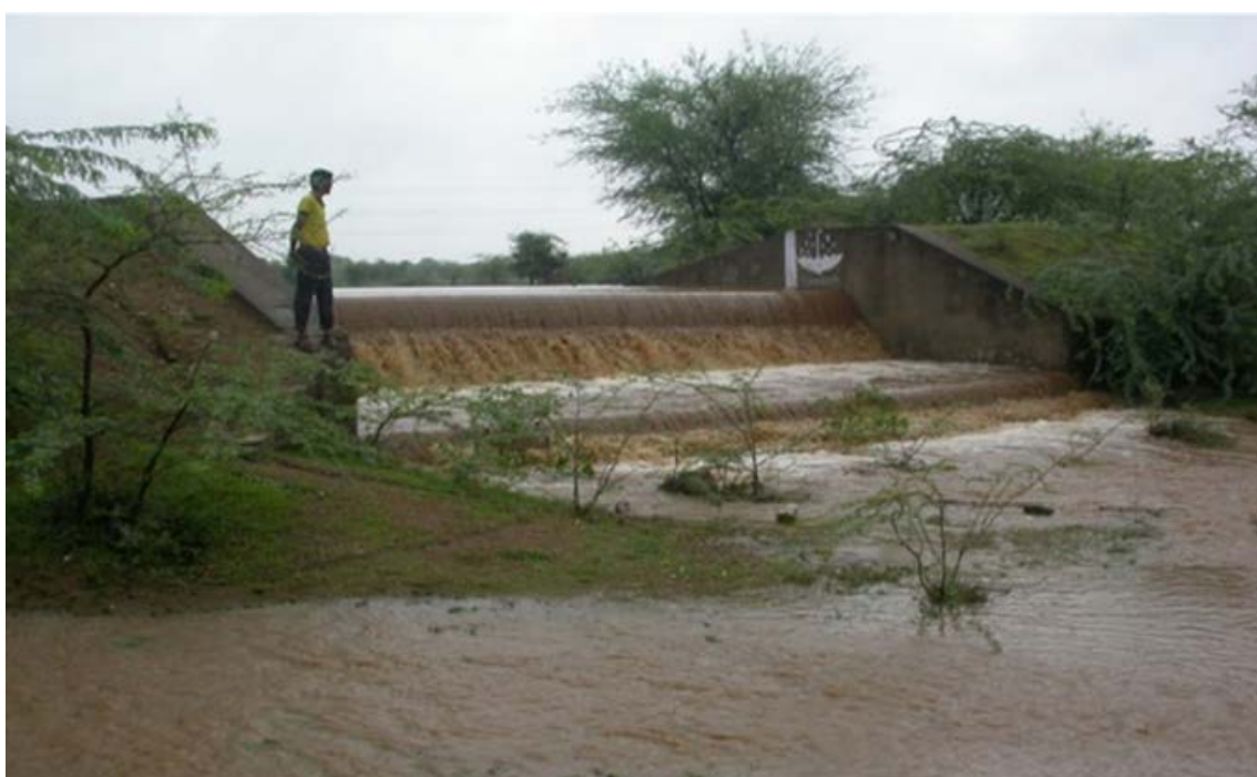
Figure 2. Badgaon check dam during a storm event. The gaugeboard is visible on the wing wall opposite. © Yogita Dashora
