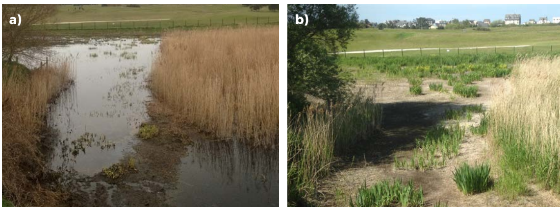
Figure 2: Central infiltration pond: a) flooded; b) dry. © Géraldine Picot-Colbeaux
