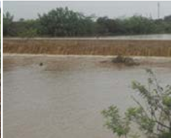
Full and spilling new check dam constructed by KVK . Baramati 2014
