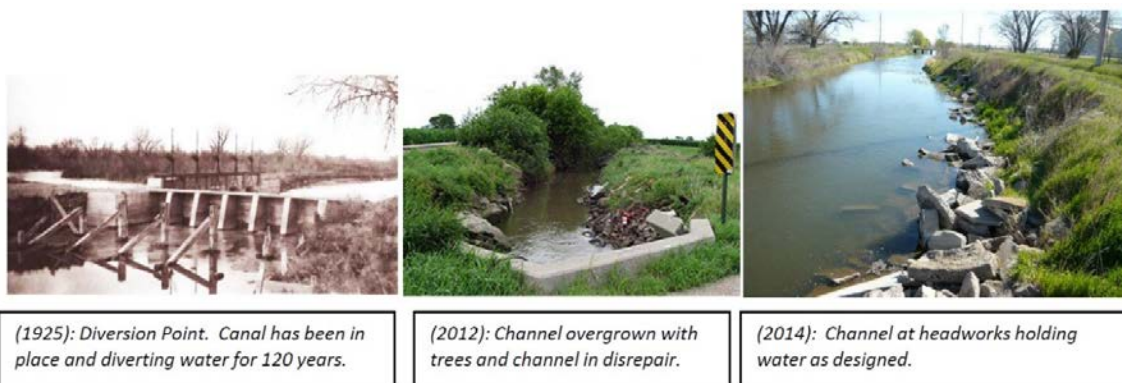
Figure 2. Historical photos of canals used in the Central Platte MAR. © Brandi Flyr
