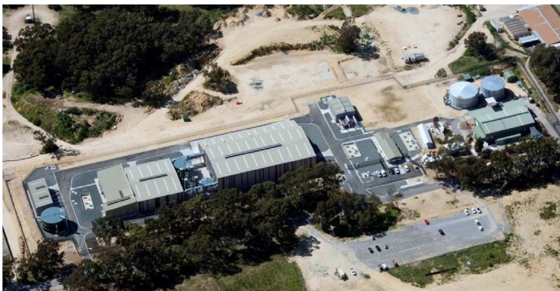
Figure 2. Groundwater Replenishment Scheme Stage 1 Advanced Water Recycling Plant. © Water Corporation of Western Australia
