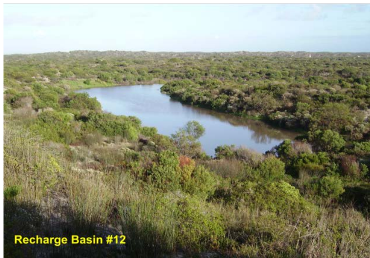
Figure 5. Recharge Basin #12 in August 2007, after a major rainfall event. The basin is mostly dry and fills only when there is sufficient peak flow storm water. Photo © chapter co-authors
