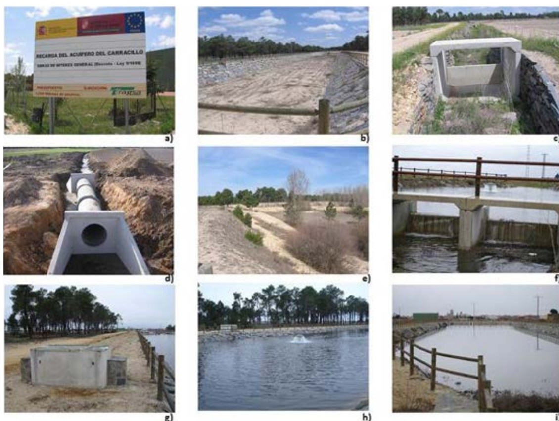
Figure 4. Components of El Carracillo MAR system: construction sign (a); Gomezserracín infiltration pond in the dry season (b); gate in a MAR canal (c); pipe for a spreading field (d); former sand pit reused as a MAR infiltration pond (e); valve and gate (Narros) (f); flow-meter to monitor the volume poured into the infiltration pond (g); Gomezserracín infiltration pond in winter season (h and i). © Jon San Sebastian
