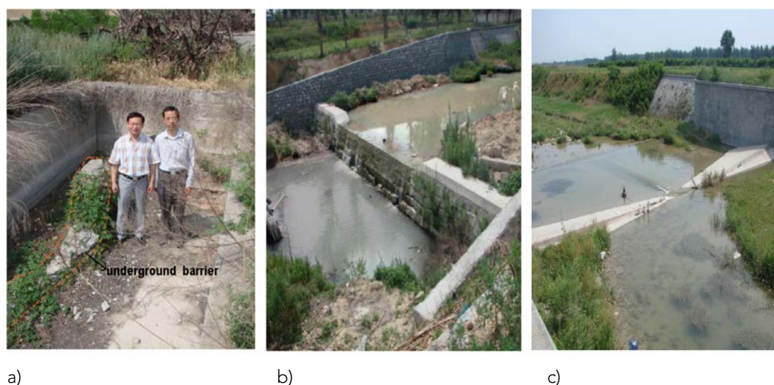
Figure 3. a) Underground dam during construction, b) weir for inflow measurement, and c) large V-shaped weir for outflow measurement. © Qingyang Zheng
